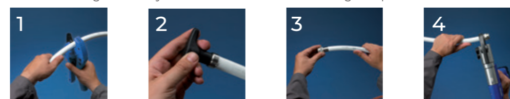
1 Couper le tube. 2 Calibrer-biseau du tube. 3 Assembler l'accessoire Tube+ Raccords. 4 Sertir - Presser.
